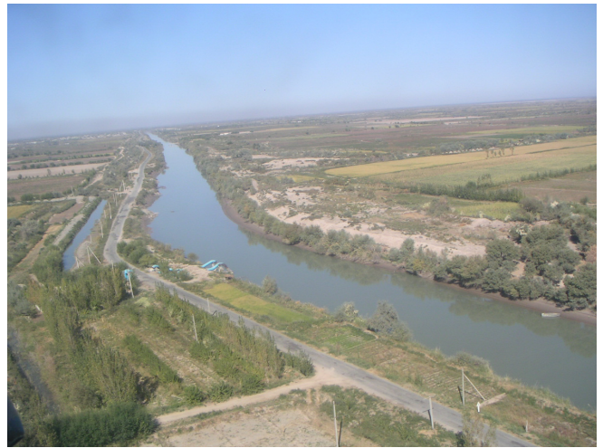
Technical improvement of water infrastructure should be combined with institutional development.
