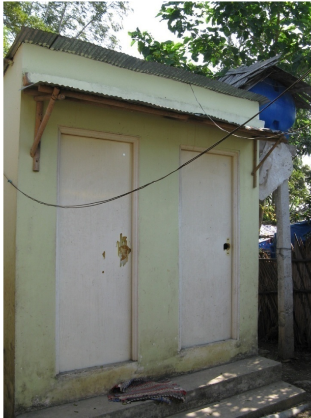
Picture 4: Septic tank latrine and bathroom
