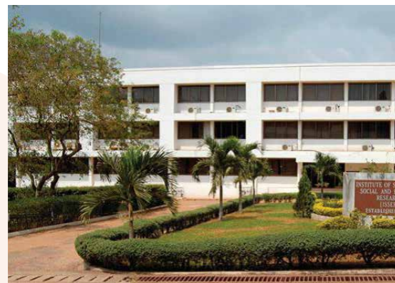
ISSER BUILDING WHICH HOUSES GGCDS
