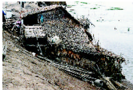
Every year, rising water levels threaten the homes along the banks of the Mekong River Photo: ZEF
