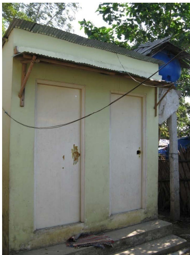
Picture 4: Septic tank latrine and bathroom
